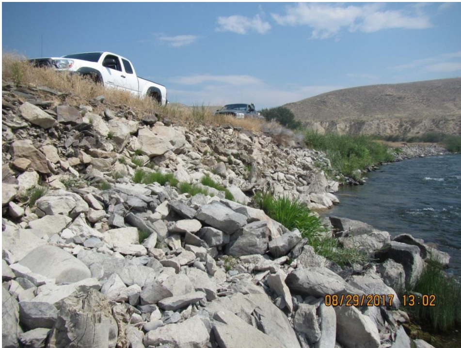
Figure 1-5: Damaged Levee Facing Upstream.
