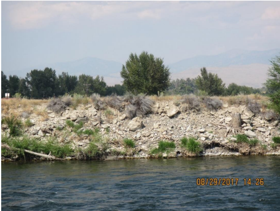
Figure 1-8: Damaged Slope on Downstream End.
