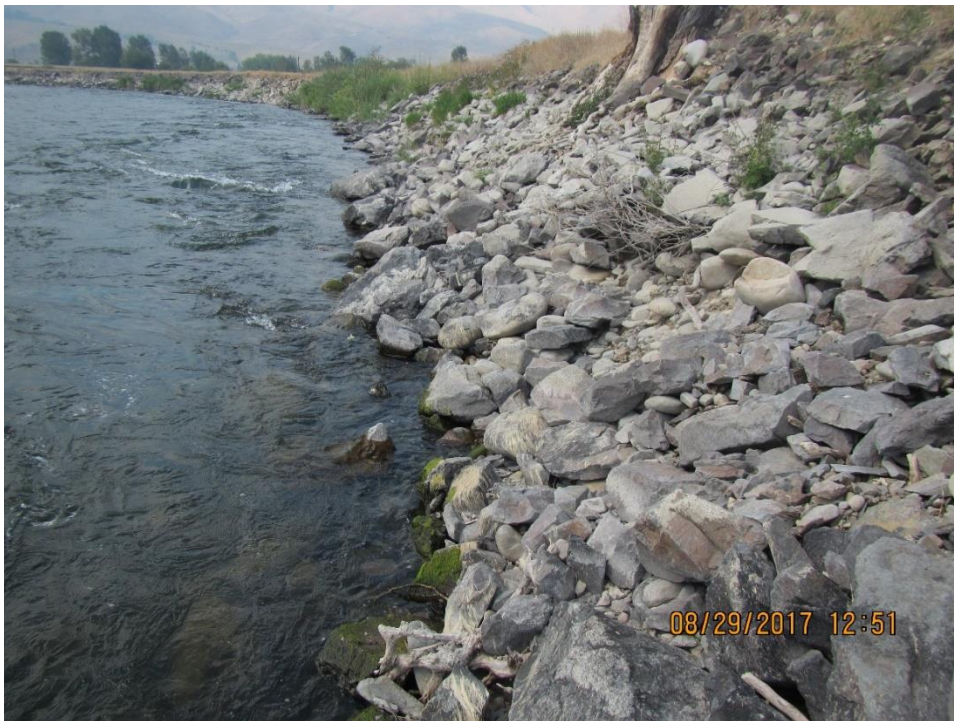
Figure 1-7: Eroded, Over-steepened Slope Facing Downstream.
